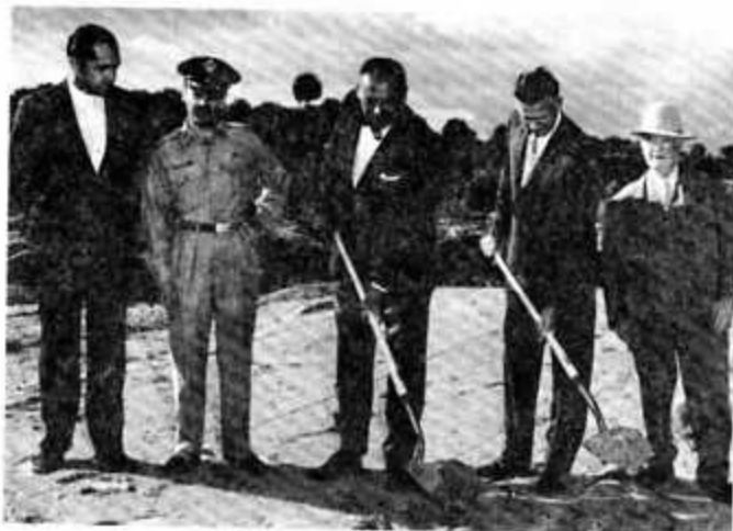
G. D. Clark, RCA-MTP Manager (right with shovel), and R. S. Mitchell, FAA-GMRD Vice President, break ground at the new FAA-RCA Building site in Cocoa Beach.
