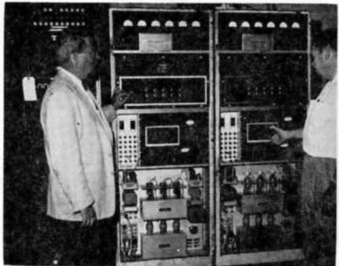
Above at left: New remote control transmitters used by the Range Safety Officer to control or destroy missiles launched from Cape Canaveral, were recently installed at range stations. Right: Installation Engineer A. K. Pooley (left) and Cape Canaveral Resident Engineer Charles Gibbs inspect the new installation.
