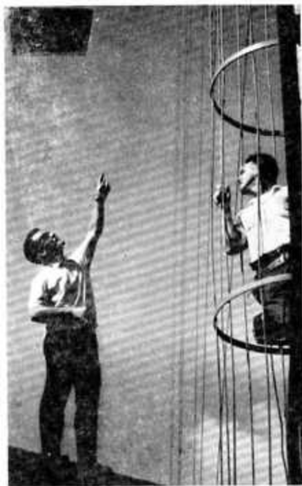
Chuck Pooley, Leader, and Tom Ball plan antenna installation on tower.
