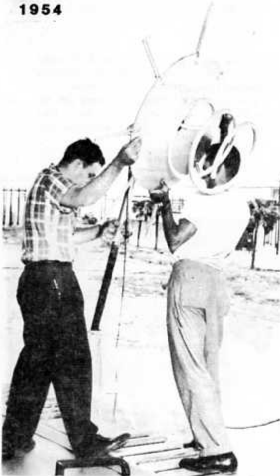
ERECTING A TELEMETERING ANTENNA on a mobile van
