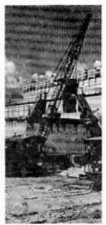
Central Control Construction
